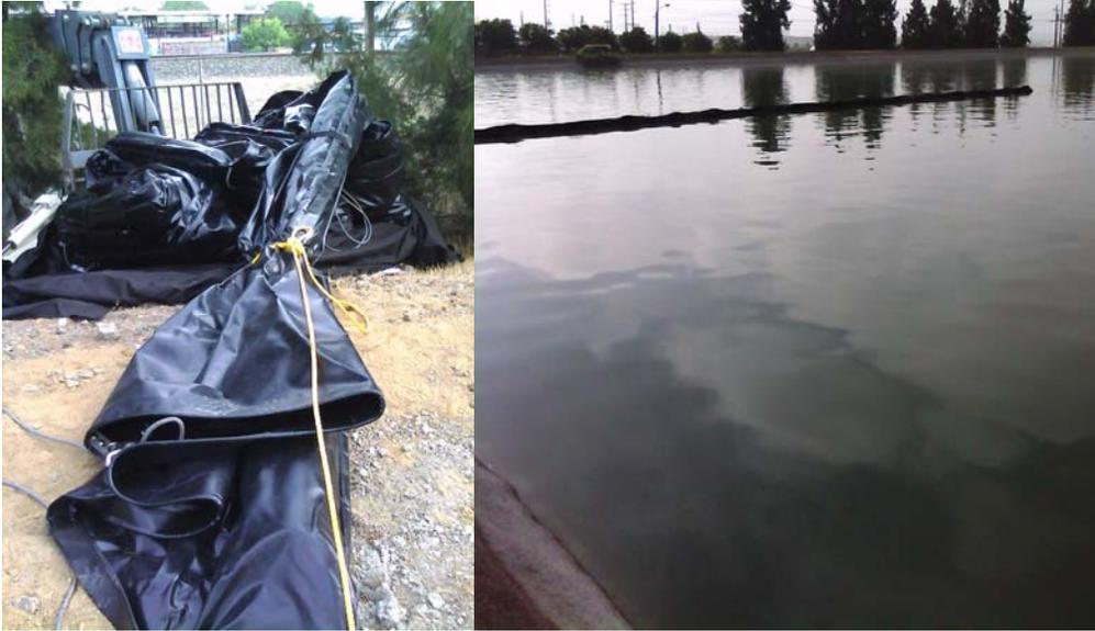
Once the floating baffle curtain was in place the bottom anchors were attached to hold the curtain in place. The result of this was a complete installation in just a day, along with a happy customer. The pond now had a longer retention time and proper flow of water.
