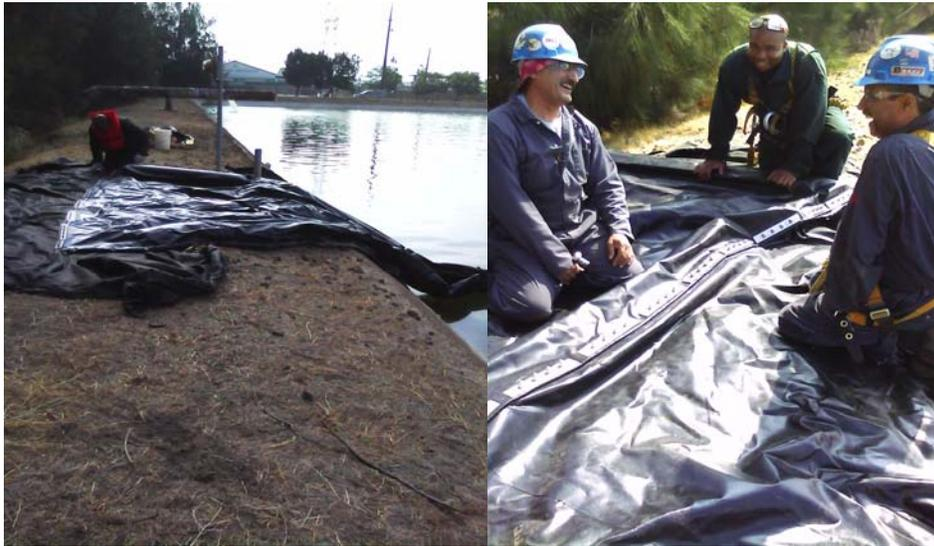
A rope was tied to the beginning section of the floating baffle curtain and placed into the water. As the curtain was placed into the pond and pulled across, it was checked for twists in the material that would prevent proper deployment. The curtain floated across into position and was attached to the shore anchor posts with stainless steel cables.
