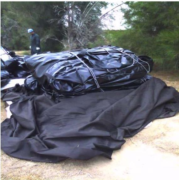
The ETP supervisor directed the installation contractor where to place the packaged baffle curtain sections for deployment. The baffle curtain was unpackaged and spread out for connecting the delivered sections together to form the complete baffle and placed at the waters edge. Once the sections of the baffle curtain were connected, the curtain was ready to be deployed into the pond.
