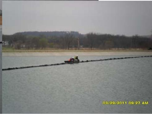
Once the floating baffle curtain was checked again for twist, the additional ballast was attached to the bottom of the curtain's skirt. The lines holding the ballast chain to the floatation collar was removed as the additional ballast was deployed which allowed the skirt to fall into position.
