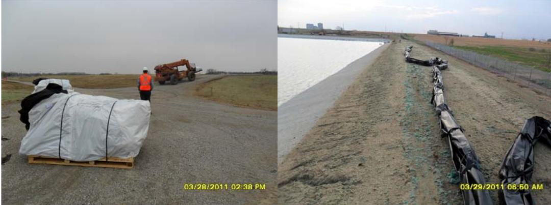
The ETP personnel directed the contractor where to place the packaged floating baffle curtain. The floating baffle curtain sections were unpackaged and spread out along the pond's berm and the bottom anchors were placed at the waters edge for easy access.
