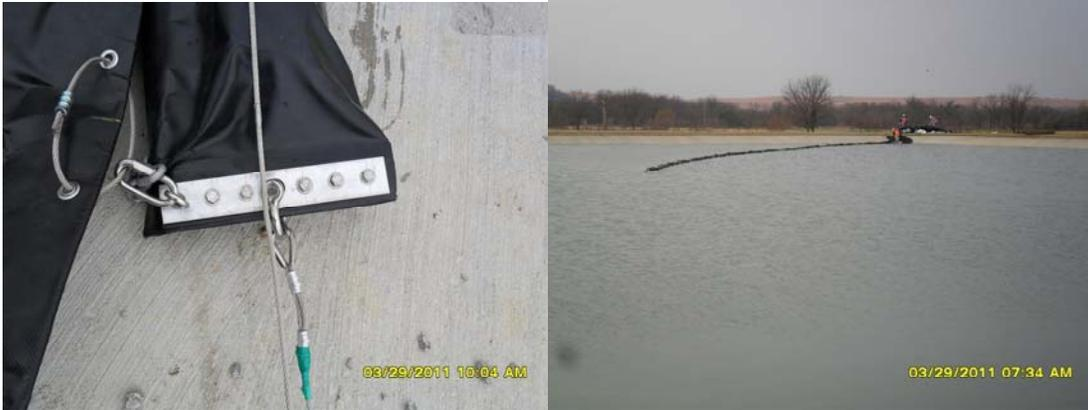
A rope was tied to the leading edge of the floating baffle curtain and then placed into the water. As the floating baffle curtain was placed into the water the floating baffle curtain was pulled across the pond using the rope attached to the leading edge.
