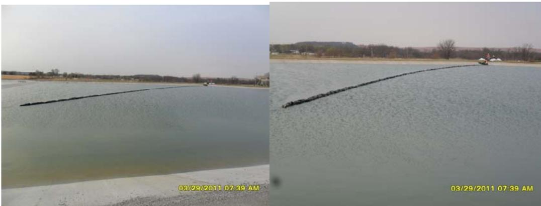
As the floating baffle curtain was pulled it floated across the pond. Once in the correct position, as shown on the project's plans the floating baffle curtain was secured to the shore anchor post.
