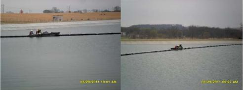
Once the floating baffle curtain was checked again for twist, the additional ballast was attached to the bottom of the curtain's skirt. The lines holding the ballast chain to the floatation collar was removed as the additional ballast was deployed which allowed the skirt to fall into position.
