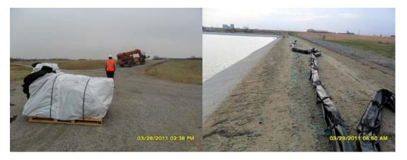
The ETP personnel directed the contractor where to place the packaged floating baffle curtain. The floating baffle curtain sections were unpackaged and spread out along the pond's berm and the bottom anchors were placed at the waters edge for easy access.
