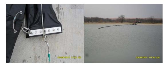
A rope was tied to the leading edge of the floating baffle curtain and then placed into the water. As the floating baffle curtain was placed into the water the floating baffle curtain was pulled across the pond using the rope attached to the leading edge.
